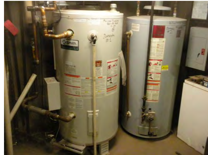
View of the two domestic hot water tanks
