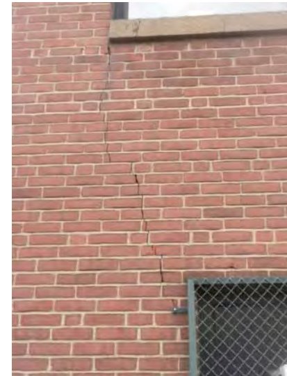
Example of cracking brick
