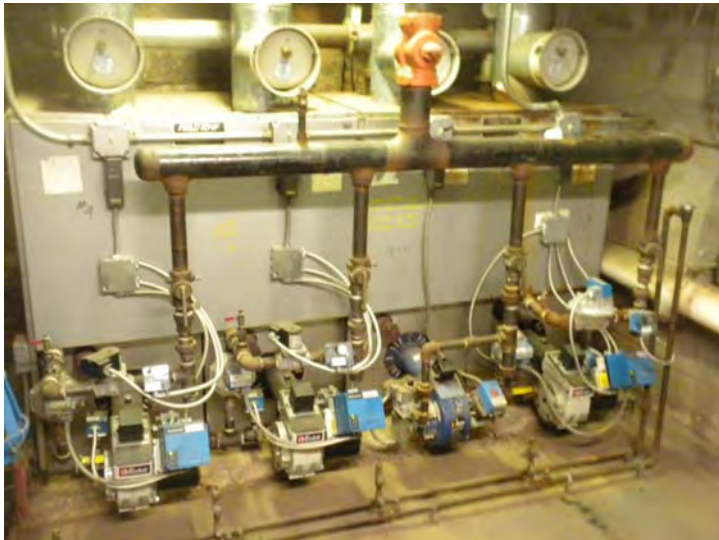
Natural gas-fired boilers
